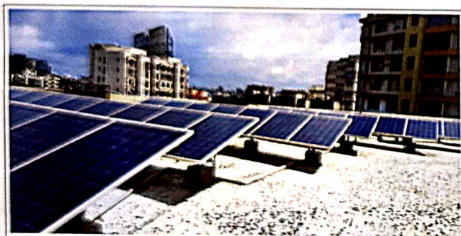
Figure 7 : Rooftop solar PV in C4 provided 20% of electricity
